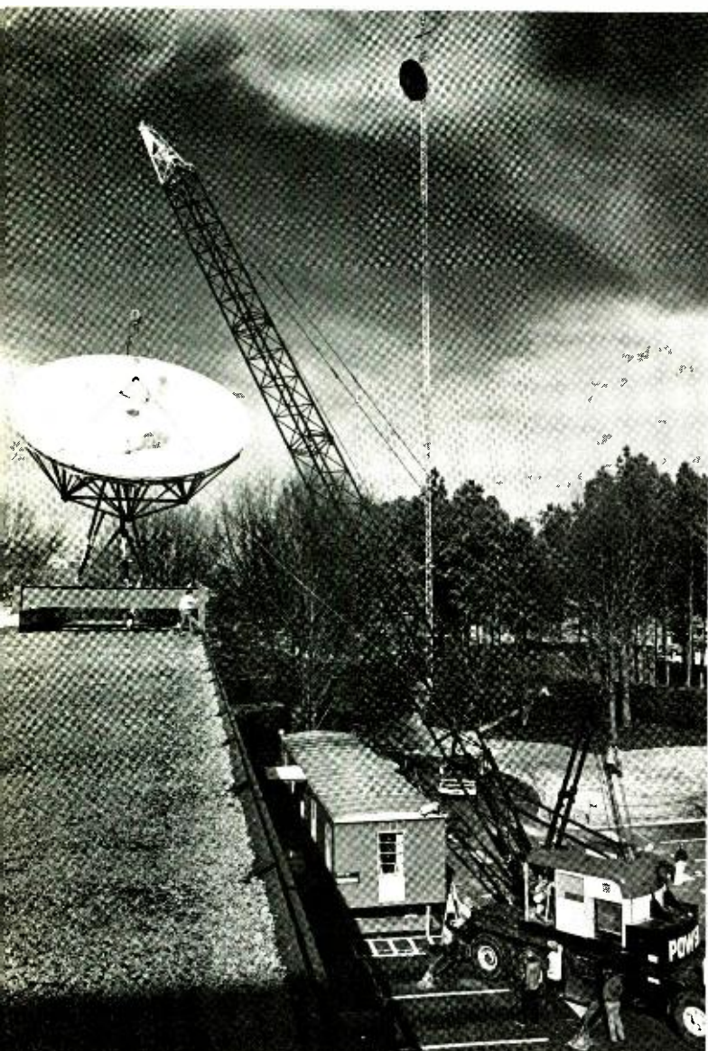
Earth terminal antenna is mounted at station WGTV, public station of the University of Georgia at Athens. The earth terminal is one of more than 200 forming PBS satellite net
