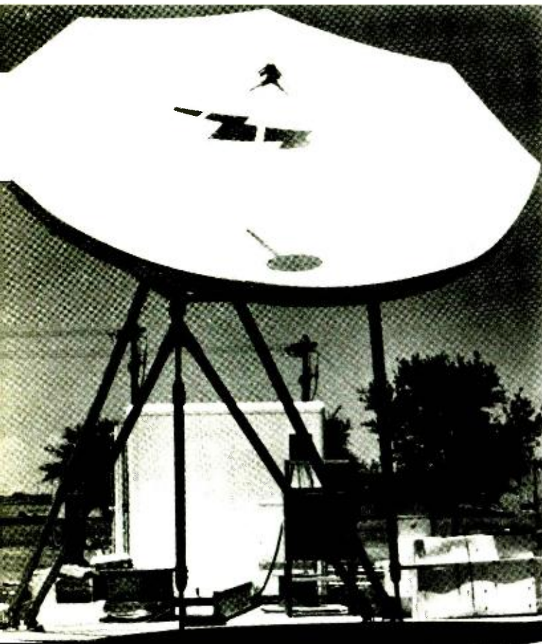
Receiving earth terminal used at National Public Radio stations on satellite net has antenna 4.5 meters in diameter, overall structure height of 20 feet. More than 200 stations have the terminals, and more are joining steadily
